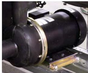
Coupled to the reservoir are centrifugal pumps to provide process flow. Single refrigeration zone chillers up to 50 tons typically use a single pump system that delivers the cooling fluid to process then returns it through the chiller's evaporator and into the reservoir.
