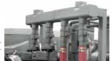
Manifold for water-cooled condensers. Manifolds include isolation valves.
